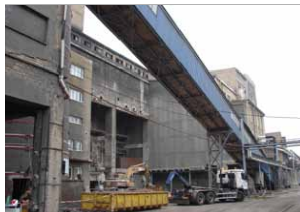
Obr. 1 Prostor demolané kotelny; 10/2013.
